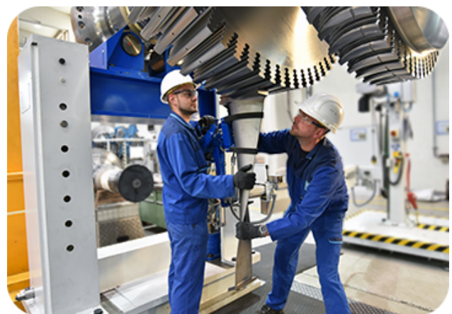
Industrial gas turbine blade being installed
